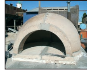
4. Place dome inner on base ensuring all connecting edges have been pre-mortared. Tap together, smooth off excess mortar from joins.
