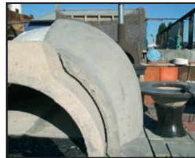
5. Ensure mantle is level with oven base when mortared in place, fit/mortar in front arch and place fibre blanket sections over inner shell.
