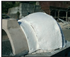
5. Ensure mantle is level with oven base when mortared in place, fit/mortar in front arch and place fibre blanket sections over inner shell.
