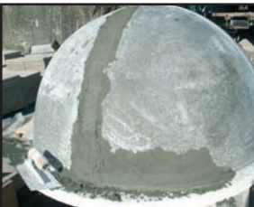
4. Place dome inner on base ensuring all connecting edges have been pre-mortared. Tap together, smooth off excess mortar from joins.
