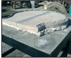
2. Oven blanket & base should be placed 200mm from edge of foundation to allow for position of mantle.
