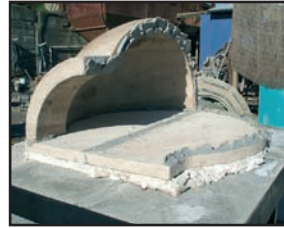
2. Oven blanket & base should be placed 200mm from edge of foundation to allow for position of mantle.
