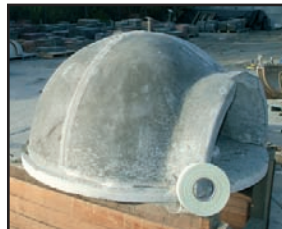
6. Place fibre tape over joints, apply cement mortar (4:1) to seal.
