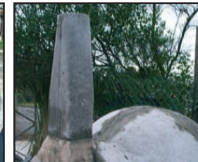
4. Place dome inner on base ensuring all connecting edges have been pre-mortared. Tap together, smooth off excess mortar from joins.
